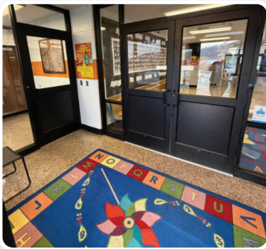
Interior of New Vestibule
